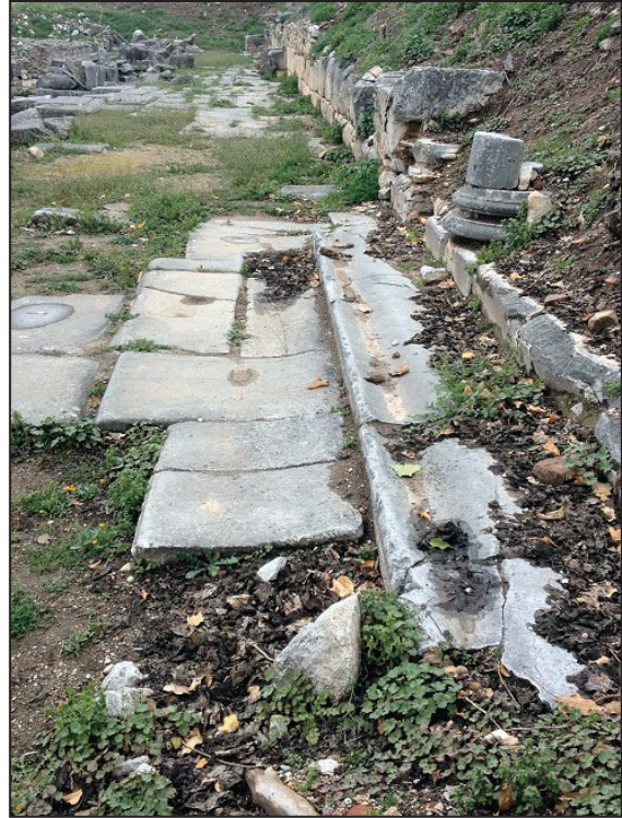
Figure 9. View of the Via Egnatia at Philippi looking west. Note the remains of an excellent gutter system to keep the road passable even in bad weather.
