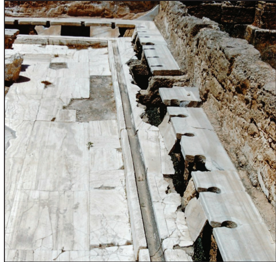
Figure 11. An impressive communal latrine located next to the public baths which could seat 60 people. It had marble seats and a deep flushing water channel under the seats. The small channel in front of the seats was used to rinse the sponges attached to sticks which served as toilet paper.
